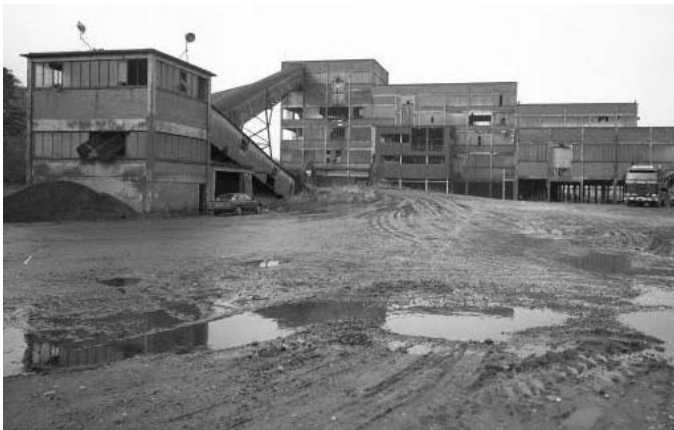
Coal preparation plant Photo © RCAHMS
