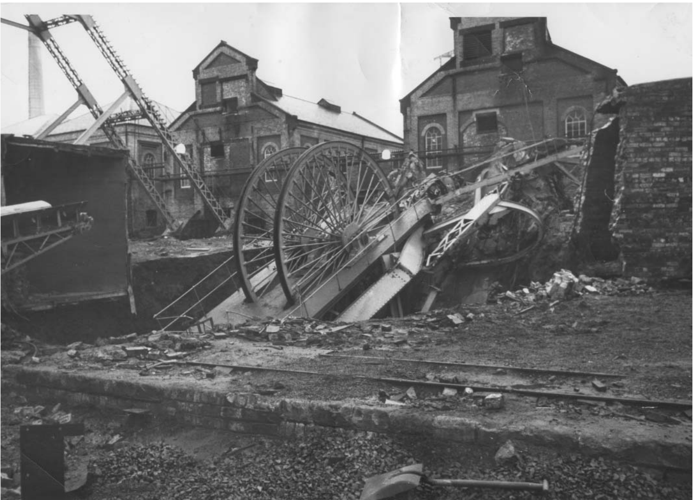
The shaft collapse Photo © RCAHMS
