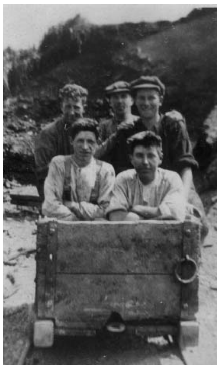
Demolition workers Photo © Mining Museum
