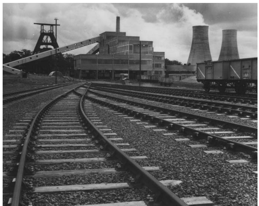
Power station at Barony Photo © East Ayrshire Libraries
